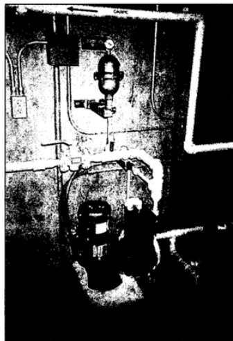
Photo 2. Metering pump installed with a pulsation dampener to inject chemicals into a process line.
